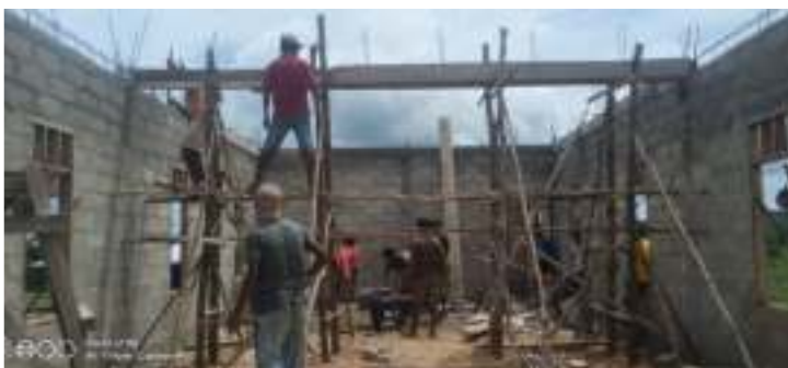
Installing the roof beam and supporting concrete cross beam
