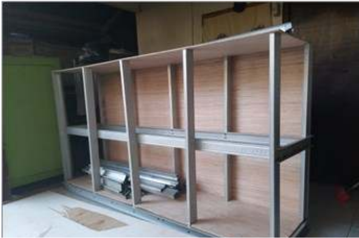
Work in progress - preparing a set of 8 new cupboard/locker/shelf units for students
