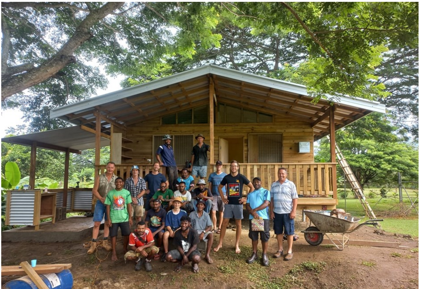
The workers responsible for erecting the 2 houses, gathered in front of house 2.
