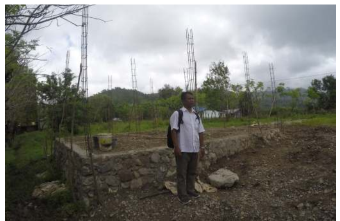
Rev. Ferdy at foundations for church at WatuBara
