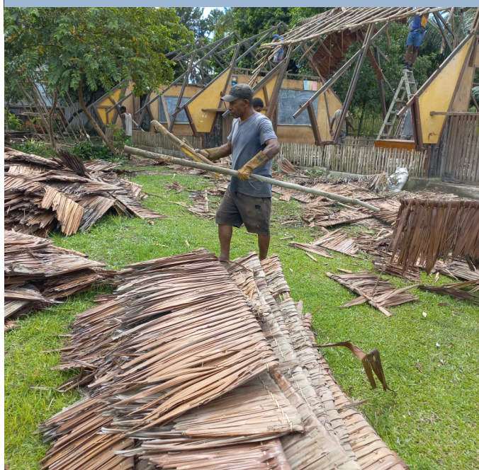
Removing the rotting morota
