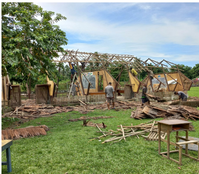
Removing the rotting morota
