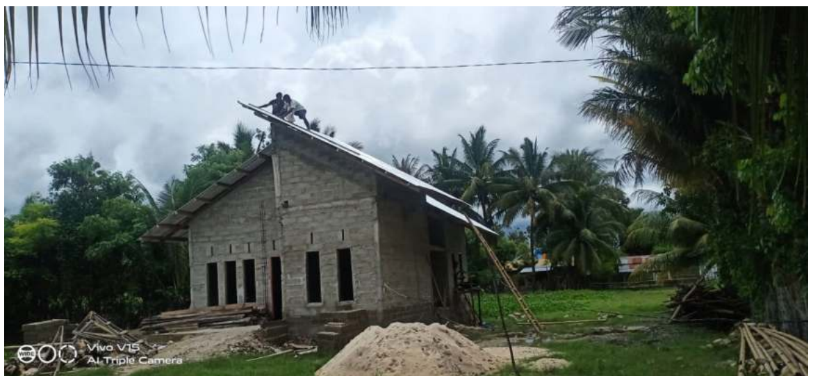
Rev Balla's new house nearing completion
