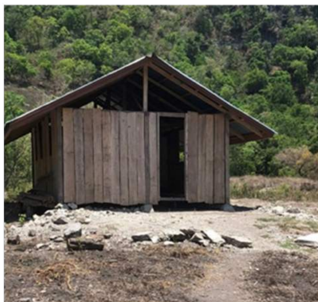
Lai Wungu Church under construction 2019
