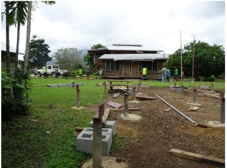
Rolling the library to its new location
